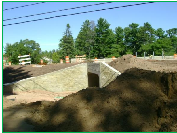
Pedestrian Tunnel Construction Summer of 2010
